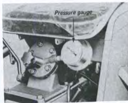
Fig. 132—To check relief pressure, a pressure gage can be installed in hydraulic cylinder head as shown.
